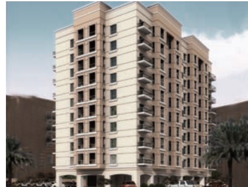
Client : Al Mazaya Real Estate Consultant : National Engineering Bureau Project : Plot 55 (G+10)
