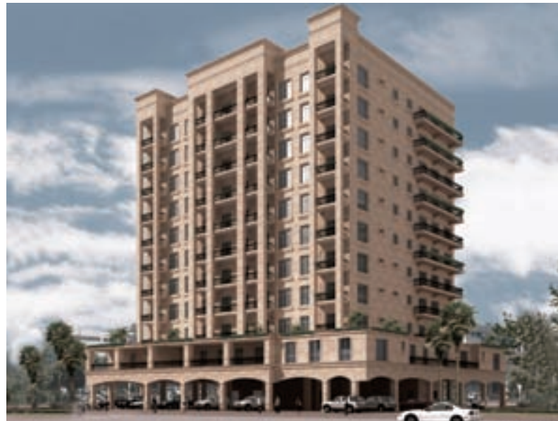
Client : Al Mazaya Real Estate Consultant : National Engineering Bureau Project : Plot 81 (G+9)
